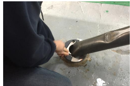
Figure 2 - Removal of Stainless Steel Cover Plates
