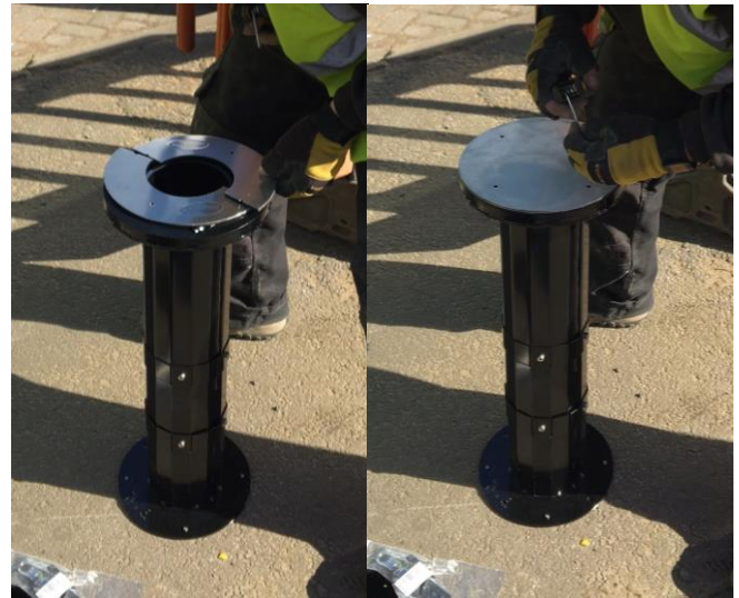
Figure 6 - Placement of Stainless Steel Cover Plates and Blanking Plate
