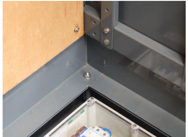
Figure 10 - M8 washer and nut used to fix cabinet to cassette and plinth, tightened to 15-20Nm.
