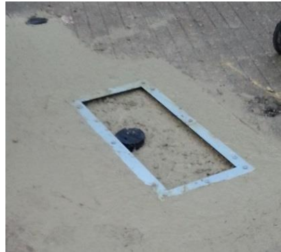
Figure 2 - After placement of ducting, the plinth is buried in concrete.
